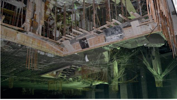
Figure 1: The collapse of the mold causing 6 people to be injured in a construction.
